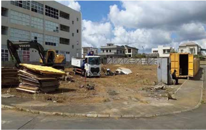
Picture 1: Removal of Vegetable Soil
