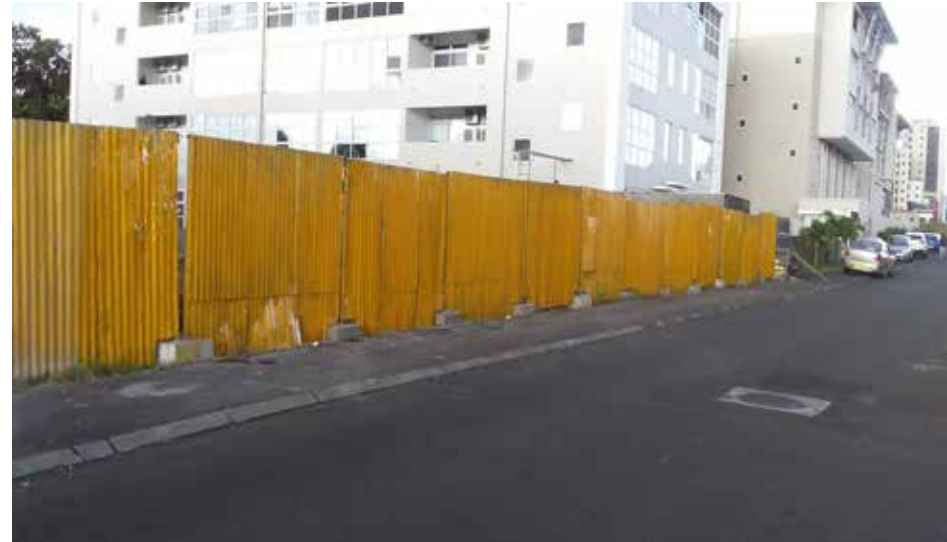
Picture 2: Fixing of Hoarding to site
