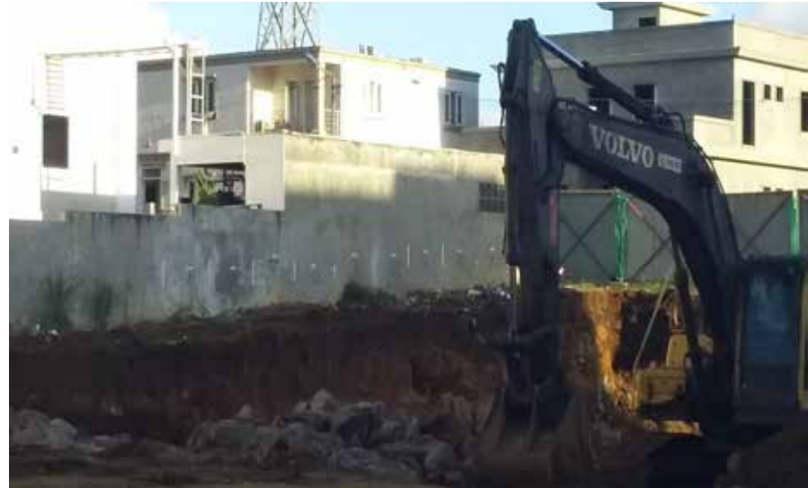
Picture 6: Setting out for underpinning works
