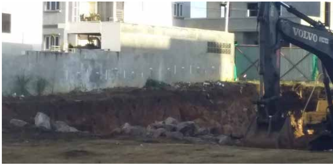
Photo 1: Setting out for first set of underpinning works
