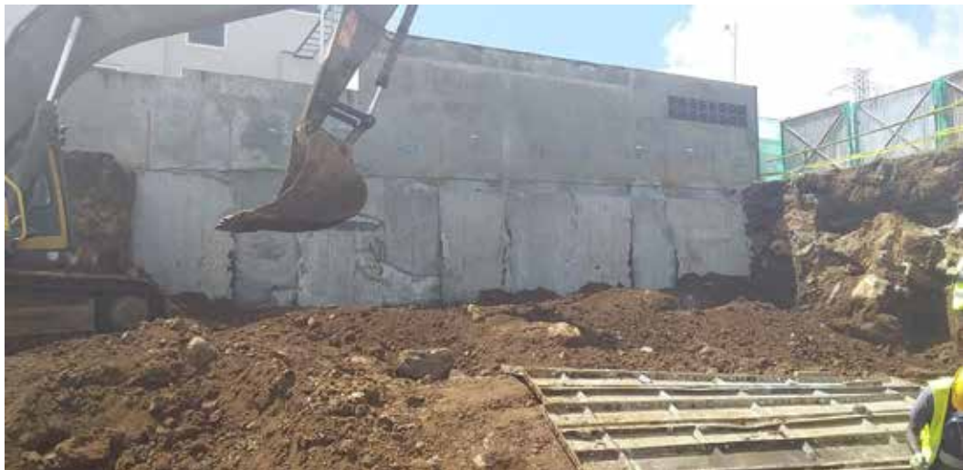
Photo 5: Casting of first set of underpinning
