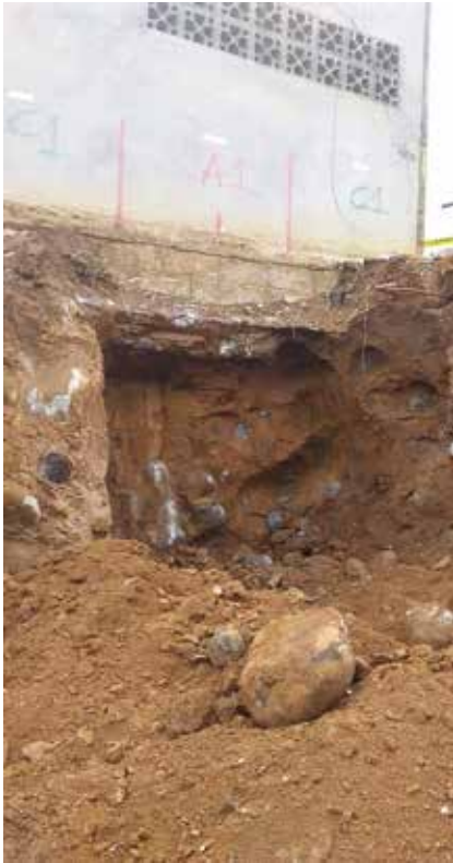
Photo 3: Excavation for first A1 pin prior to propping and shuttering
