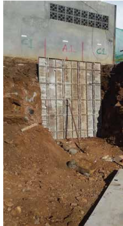
Photo 4: Shuttering to first A1 pin
