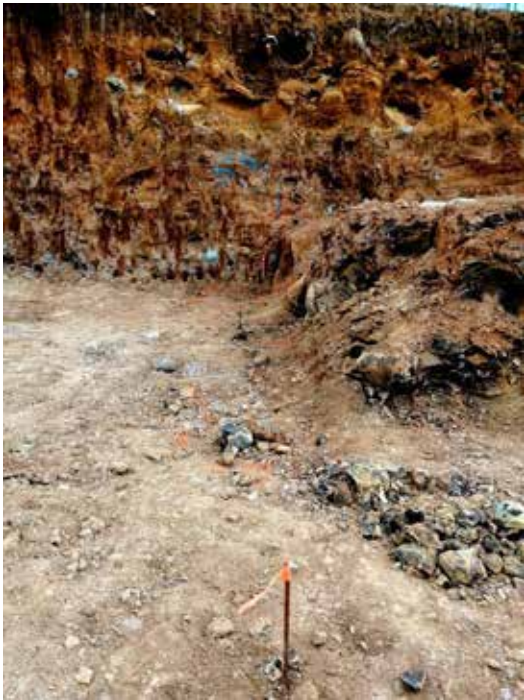
Photo 7: Setting out for column bases and retaining wall base
