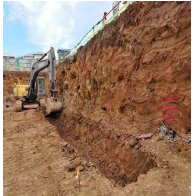
Photo 8: Excavation to formation level for retaining wall base
