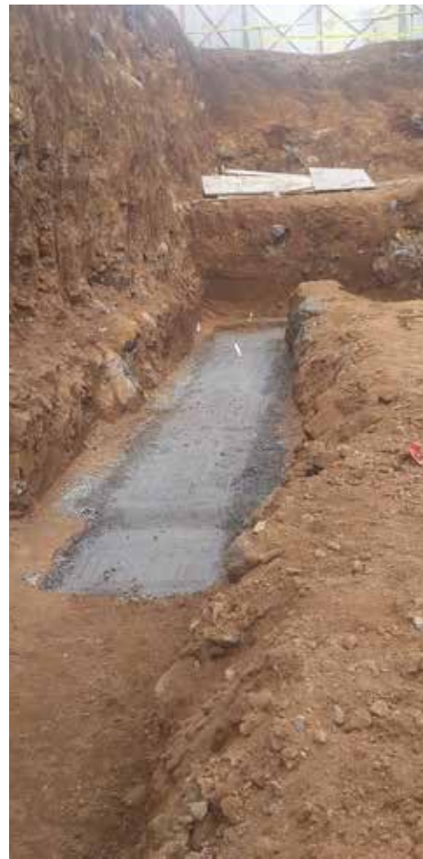
Photo 3: Casting of blinding along GL k'/1-4
