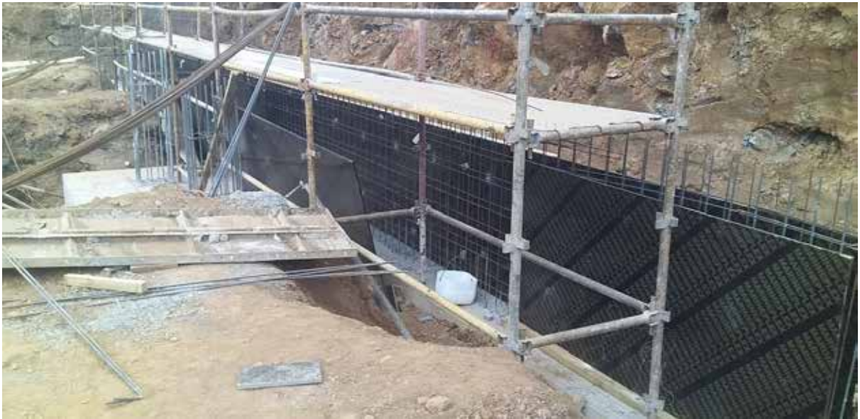
Photo 7: Shuttering to retaining wall along GL E-K'/7'
