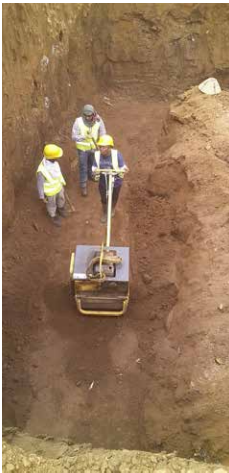
Photo 2: Compaction to sub base prior to laying of blinding
