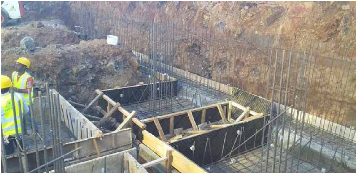
Photo 5: Formwork and Reinforcement to column bases and starter bars for columns
