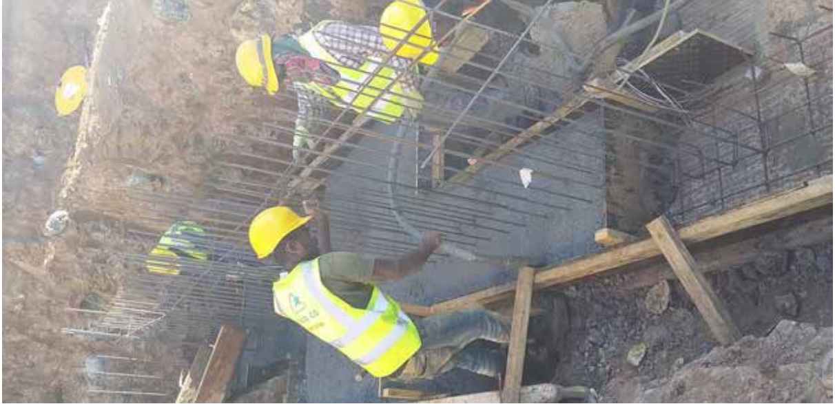
Photo 6: Casting to retaining wall base and column bases along GL J-K'/4
