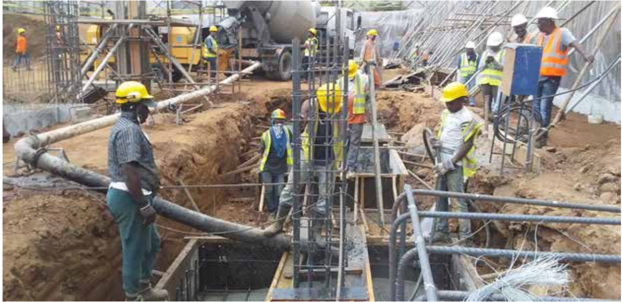
Photo 6: Casting to column bases at GL F-H/1
