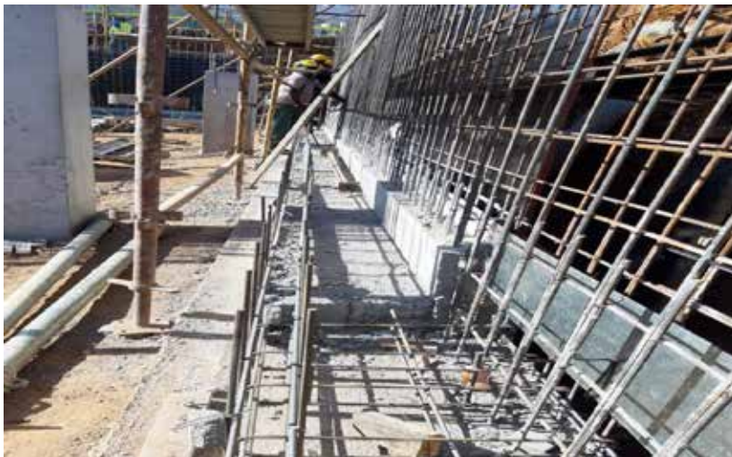
Photo 3: Drain along GL E-J/7'
