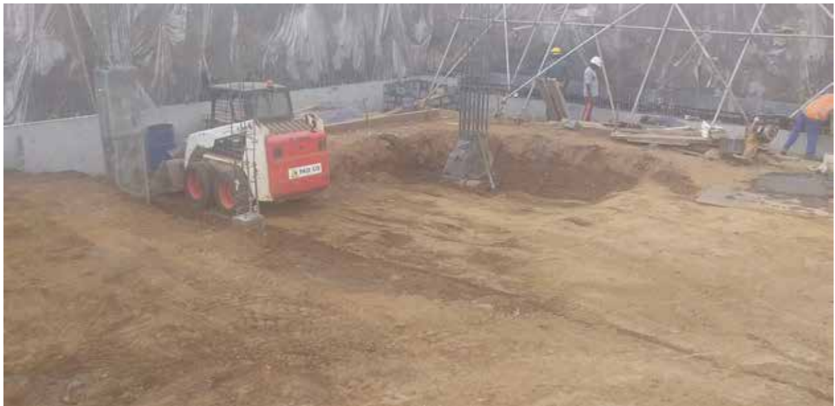
Photo 10: Selected fill & Compaction prior to laying of spalls
