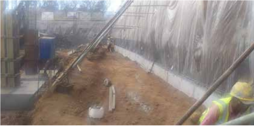
Photo 1: Selected fill & compaction below drain
