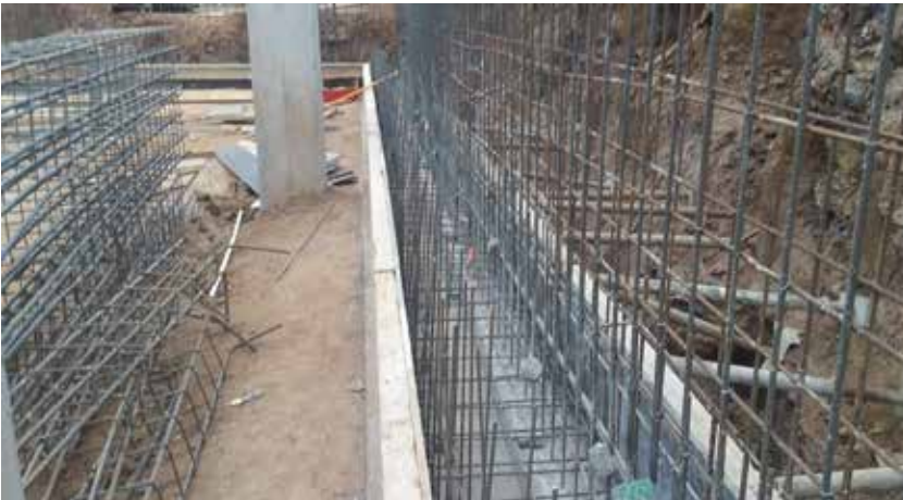
Photo 2: Reinforcement, water bar and boxing to drain along GL E-J/7'
