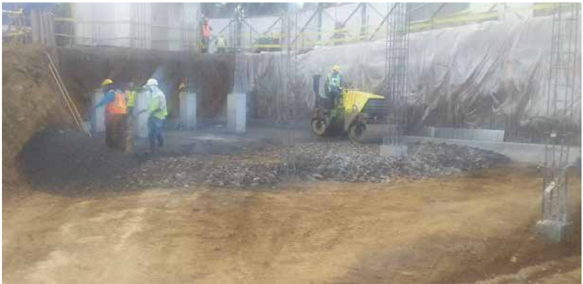
Photo 5: Laying of spalls and crusher run to floor between GL A'-Ax/3-7'
