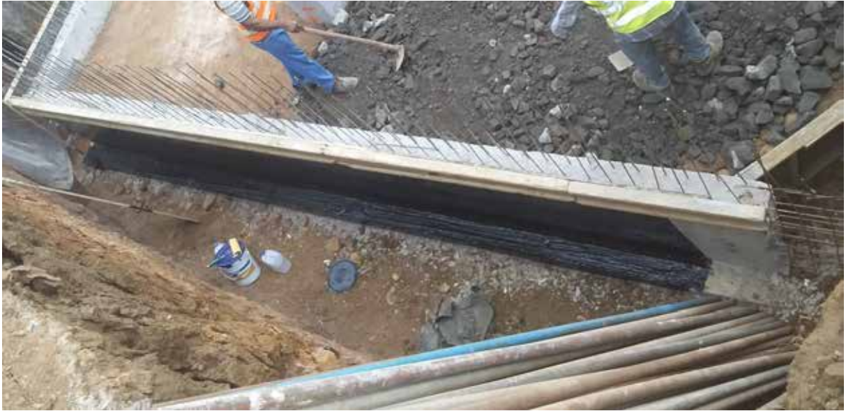
Photo 4: Laying of tanking membrane to retaining wall along GL A-Ax/7'
