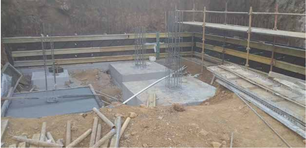
Photo 7: Shuttering to retaining wall along GL A-AX/7' and casted columns between GL 3-6
