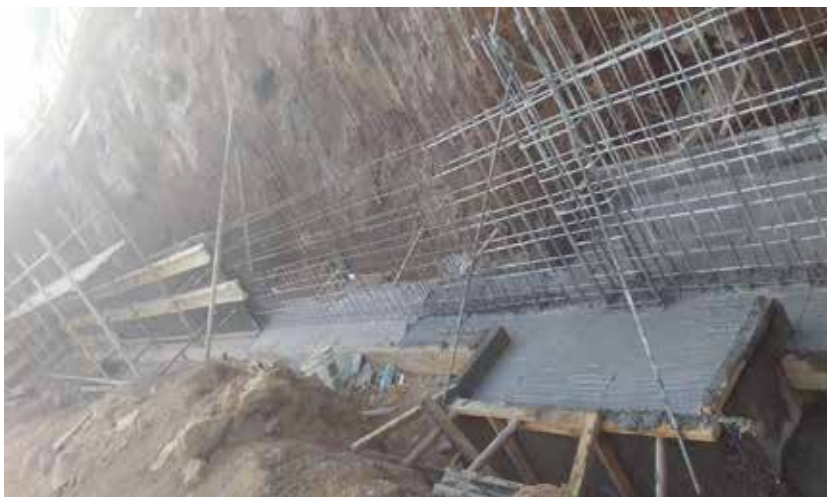
Photo 3: Casting to retaining wall base and column base along GL 1'
