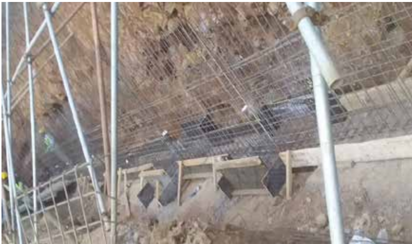
Photo 2: Reinforcement to retaining wall and retaining wall base along GL 1'/A-E
