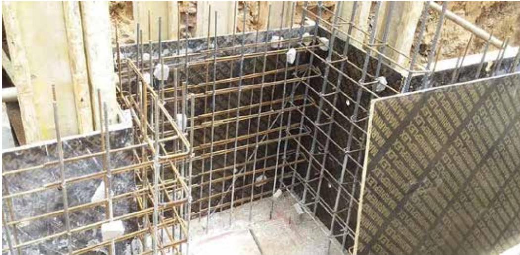
Photo 4: Formwork and Reinforcement to retaining wall along GL J/4-7'
