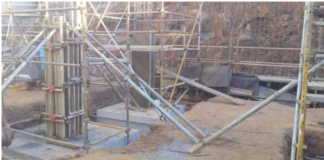
Photo 6: Casting to retaining wall base and column bases along GL J-K'/4
