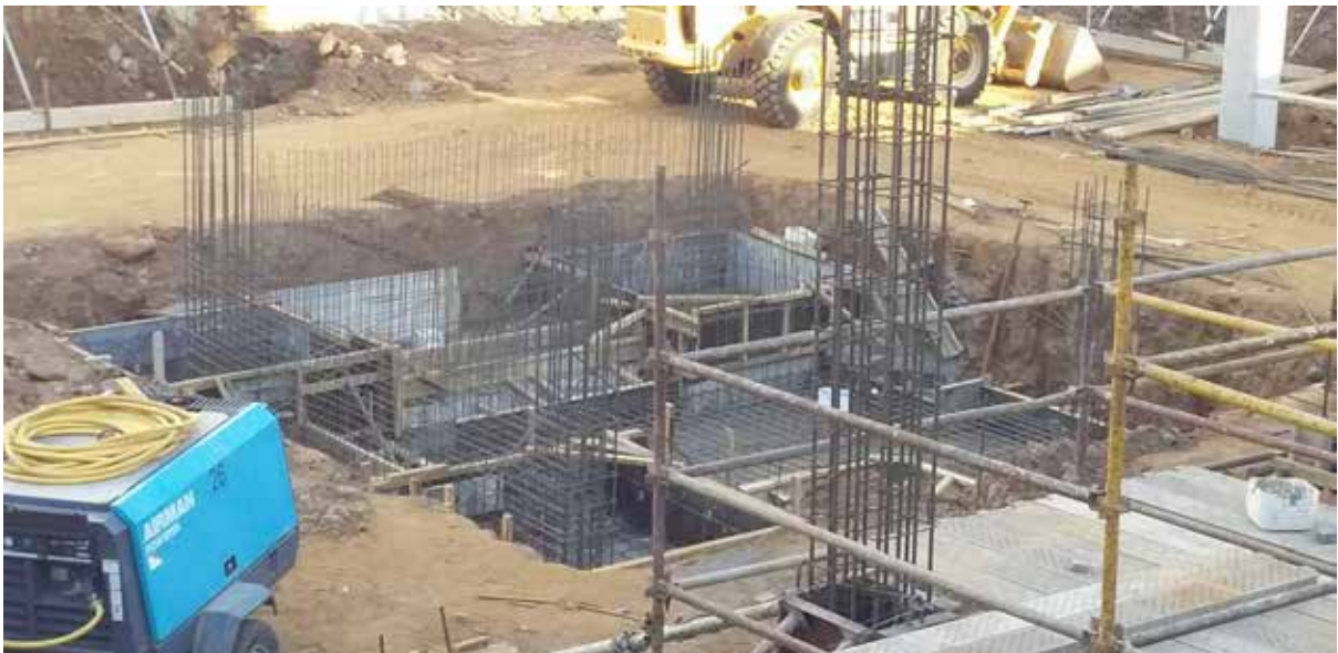
Photo 7: Shuttering to retaining wall along GL A-AX/7' and casted columns between GL 3-6
