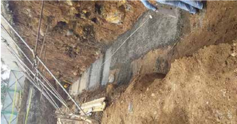
Photo 1: Casting of blinding along GL 1'/A-E
