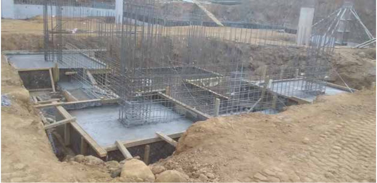
Photo 9: Casting of column bases at lift pit
