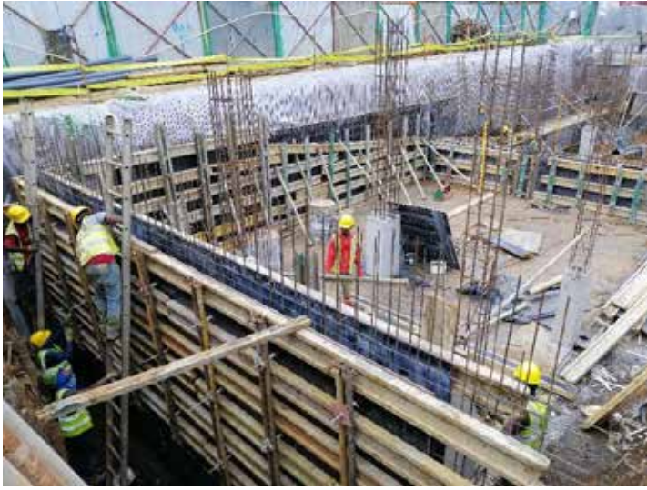
Photo 9: Reinforcement and shuttering to retaining wall along GL A'-AX/1-7'
