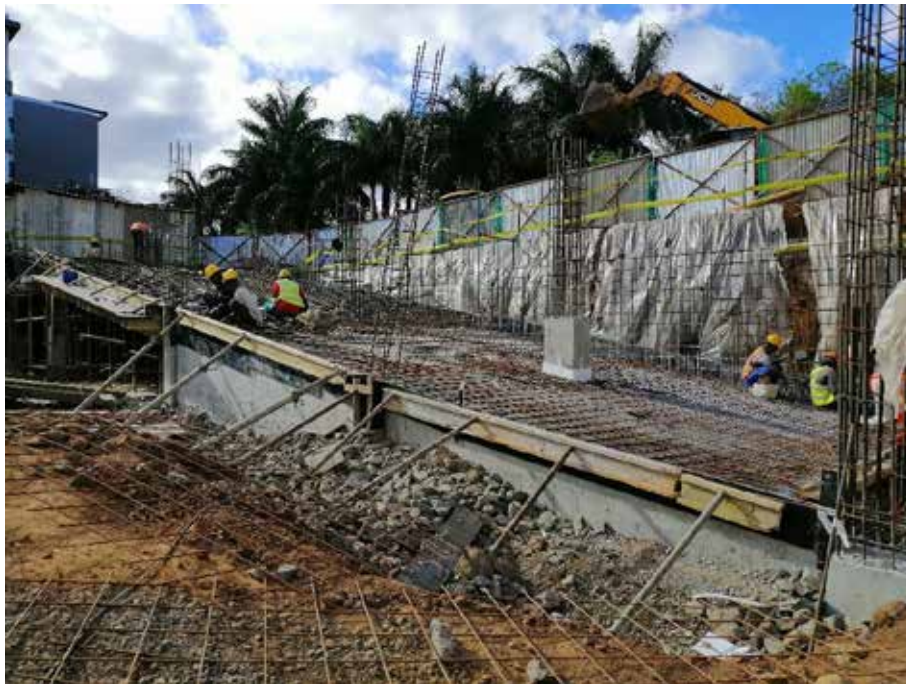
Photo 11: Reinforcement & Shuttering to Ramp 2 along GL A'-AX/1-7'
