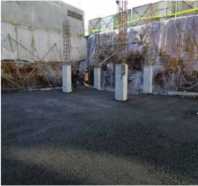
Photo 5: Compaction of crusher run along GL H'-K'/1-2'
