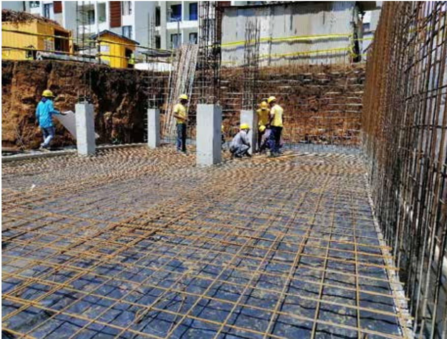
Photo 3: Reinforcement to Basement Floor B2 along GL A'-AX/3-7'
