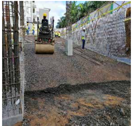
Photo 10: Compaction of crusher run along GL A'-X/1-2'
