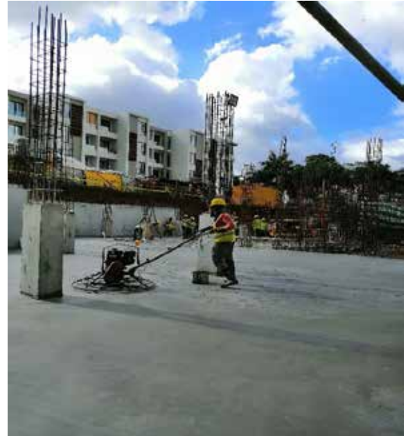
Photo 8: Power Floating floor of Basement B2 along GL H'-J'/1-2'
