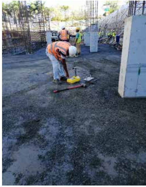
Photo 6: Compaction of crusher run along GL H'-K'/1-2'
