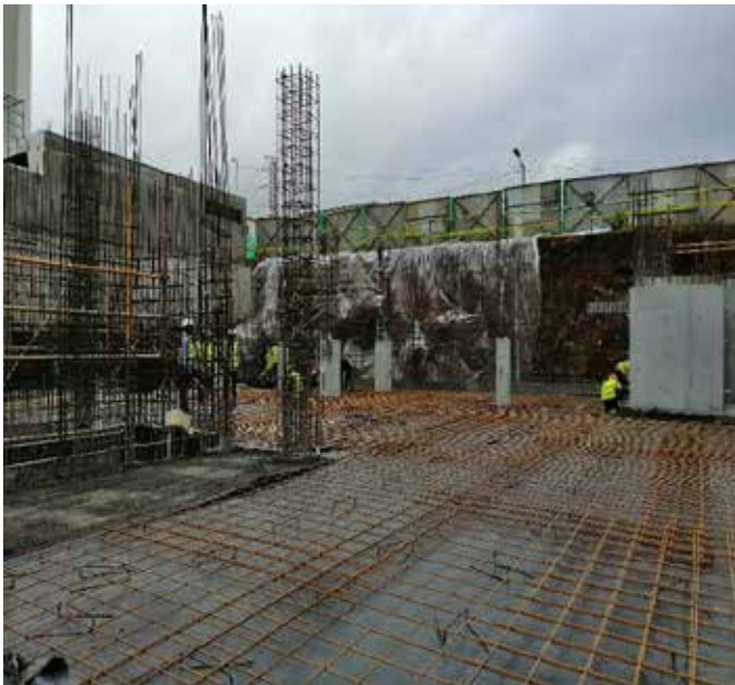
Photo 7: Reinforcements to Basement Floor along GL F'-K'/1-3'
