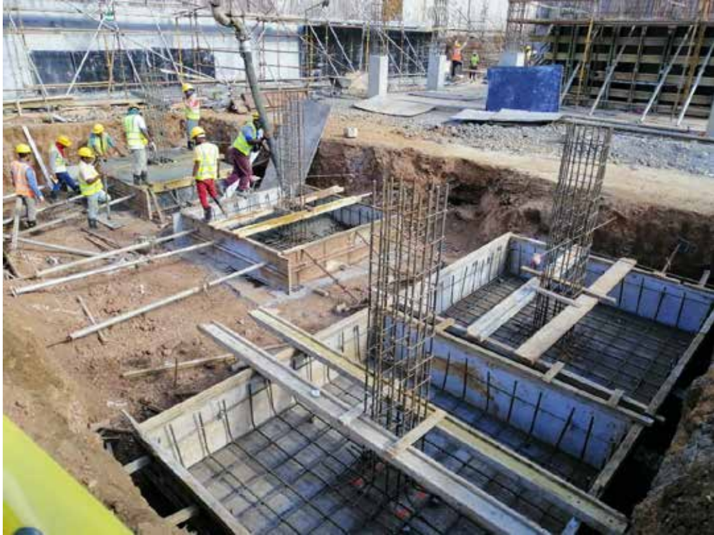
Photo 12: Casting of bases E-1, E-2, E-3 & D-3
