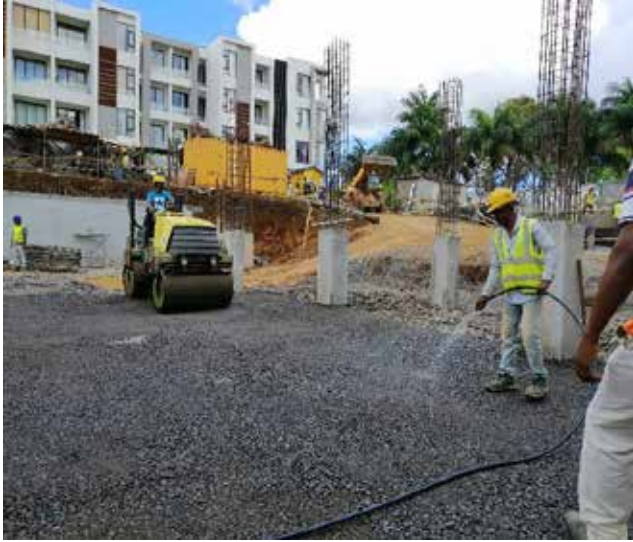
Photo 7: Compaction of crusher along GL D-F/1'-7
