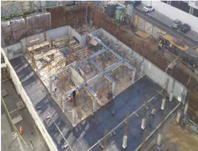
Photo 9: Reinforcement to Basement Floor B2 along GL D-F/1'-7 & GL F-K/1'-1
