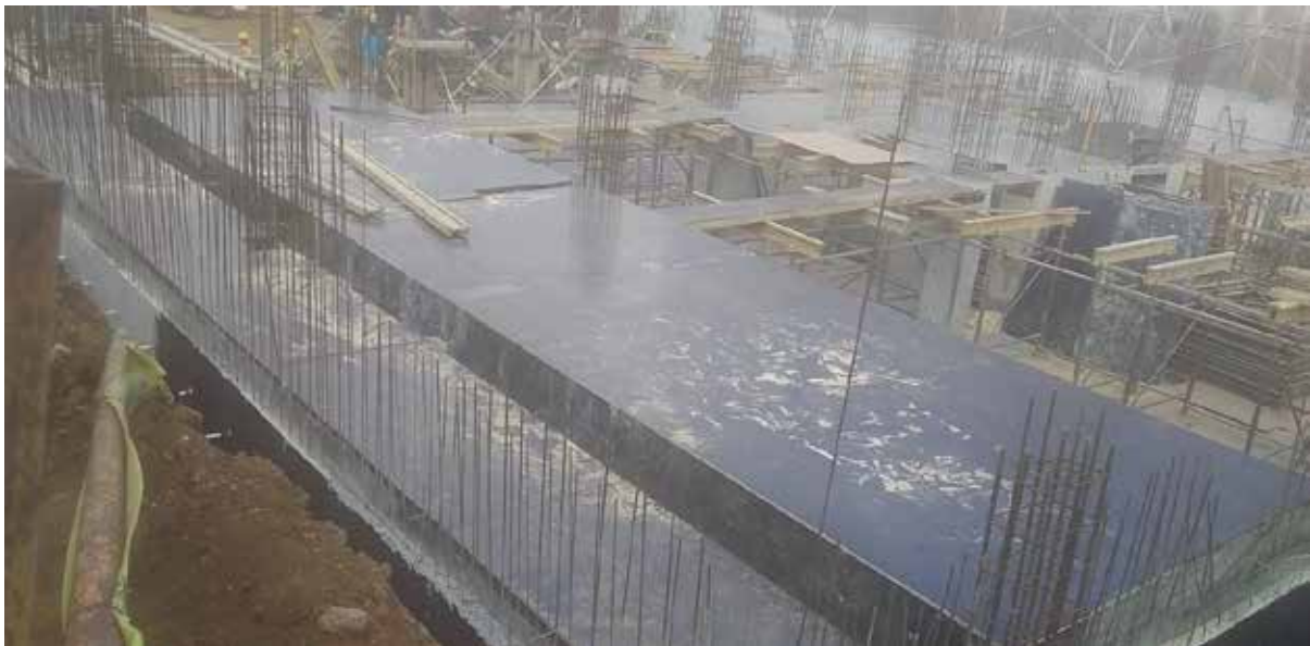
Photo 12: Formwork to slab and side drain
