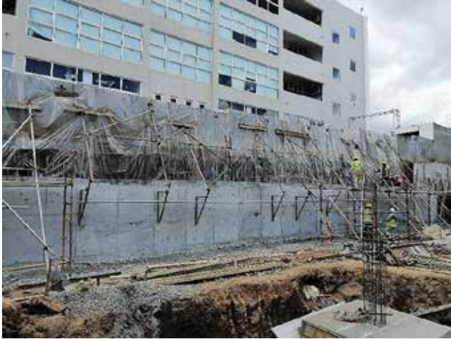
Photo 1: Knee bracing against Catéco wall
