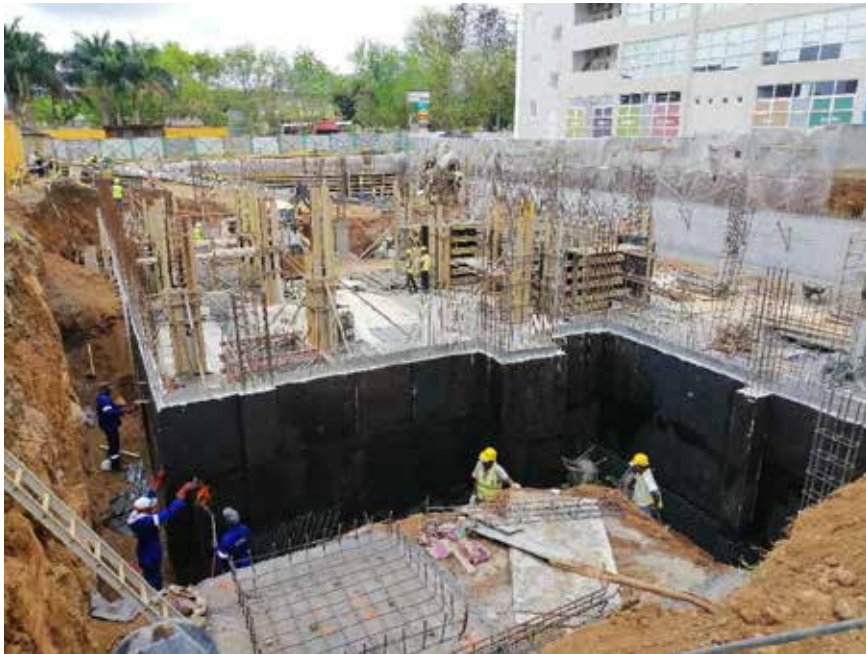
Photo 3: Installation of tanking membrane along GL J/7
