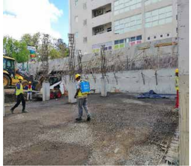
Photo 8: Anti-termite treatment along GL D-F/1'-7
