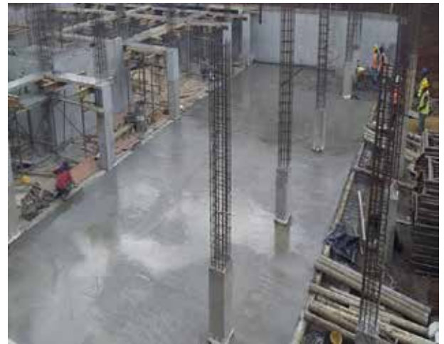
Photo 10: Casting of Basement Floor B2 along GL D-F/1'-7
