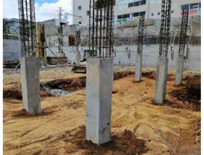
Photo 2: Backfilling across GL D-E /1-3'
