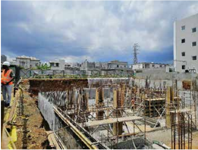
Photo 4: Formwork to stub columns and lift shaft along GL G-J /1-6
