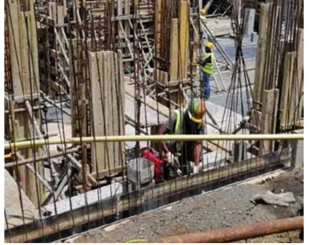
Photo 5: Installation of water bar at GL D-E /7
