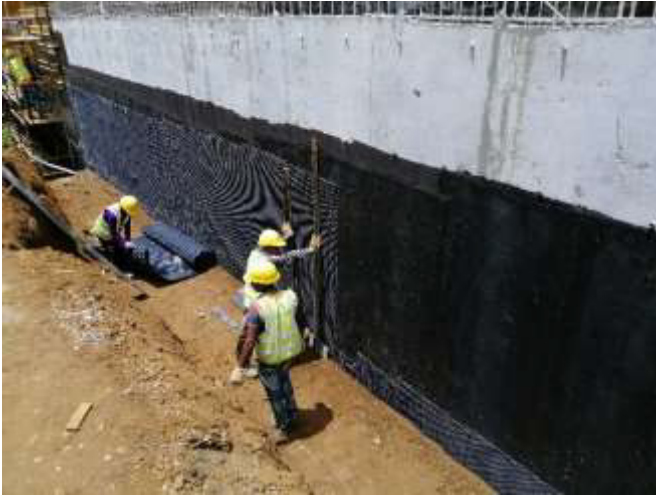
Photo 13: Application of protection to tanking membrane at GL D-F|7
