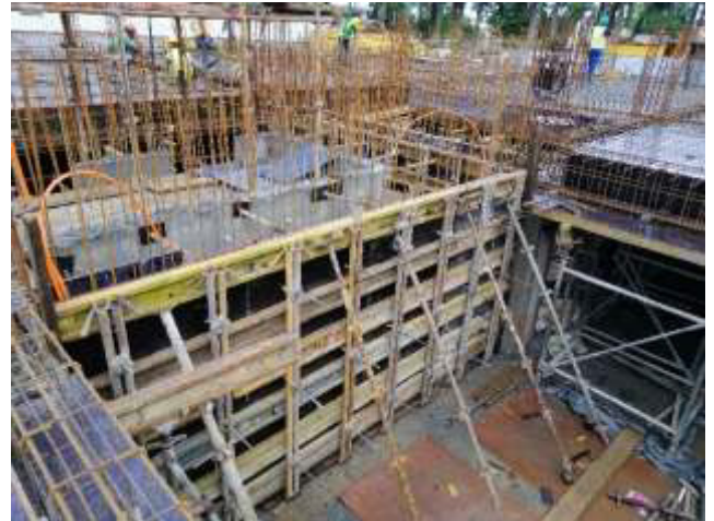
Photo 10: Shuttering to reinforcement at staircase 1 along GL G-H|2-3
