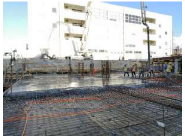
Photo 4: Casting of Basement B1 floor slab
