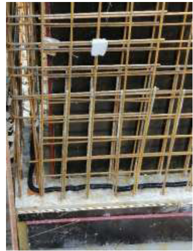
Photo 14: Installation of penebar to water tank reinforcements
