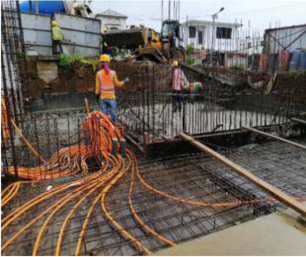
Photo 5: Casting of Water Tank floor slab at Basement B1
