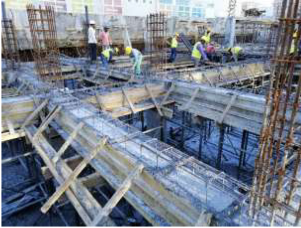
Photo 1: De-shuttering of beams at GL Ax-D' | 1-6
