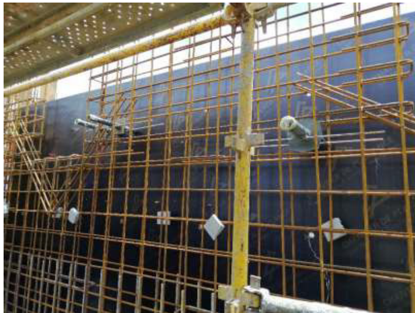
Photo 15: Installation of puddle flange at water tank
