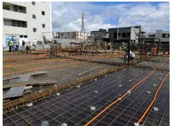
Photo 12: Reinforcement to formwork and installation of conduits for Basement B1 slab
