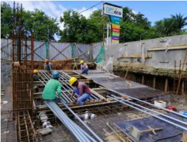
Photo 7: Shuttering to Ramp 1 at GL A-Ax|1'-1
