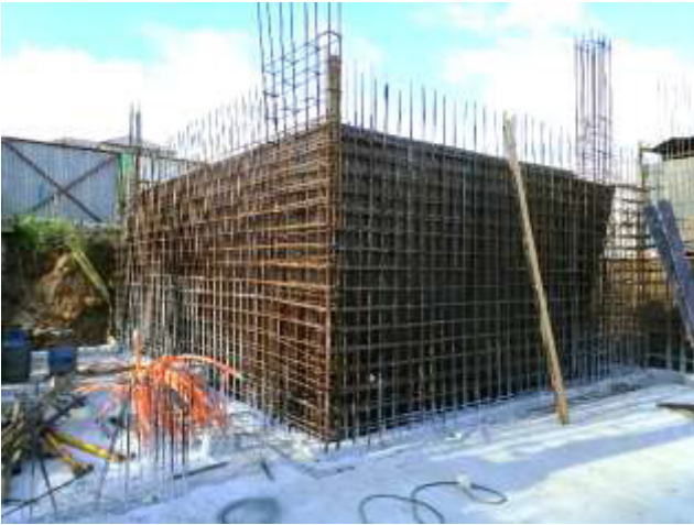
Photo 9: Shuttering to reinforcement for wall at water tank along GL J-Kx|4-7
