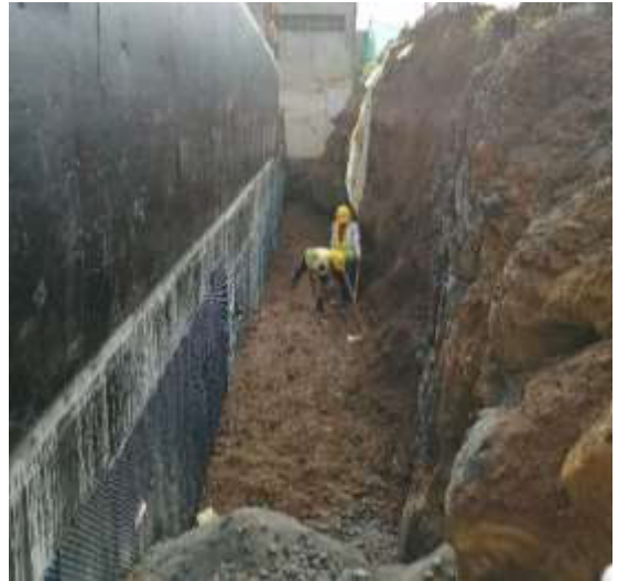
Photo 6: Backfilling at GL Kx|1-4
