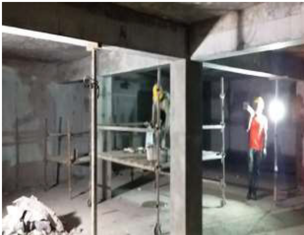
Photo 11: Rendering of columns and beams at Basement B2 along GL K-Kx|2-4
