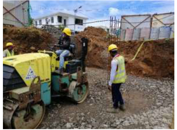
Photo 2: Compaction of spalls at water tank area along GL J-Kx | 4-7
