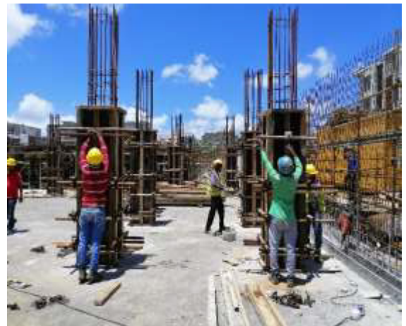
Photo 8: Shuttering to column reinforcement at GL C-D|5-6
