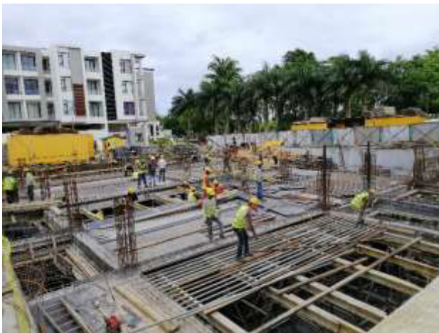
Photo 3: Shuttering to Basement B1 floor slab and beams along GL Ax-D' | 1-7
