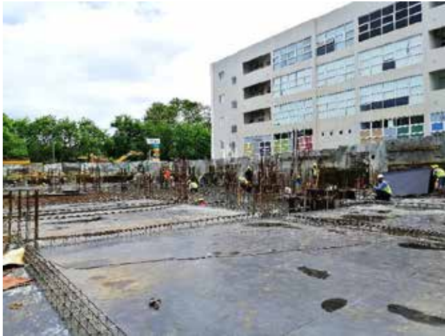
Photo 10: Shuttering of Basement B1 floor slab
