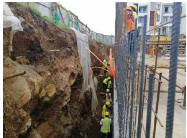
Photo 15: Backfilling and reinforcement to retaining wall at GL K'|1'-4
