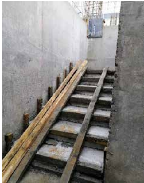
Photo 3: Casting of a section of staircase at GL G-H |2-3
