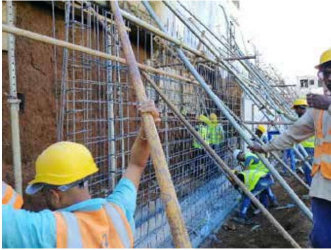
Photo 1: Additional vertical support carried out below boundary wall of Cateco
