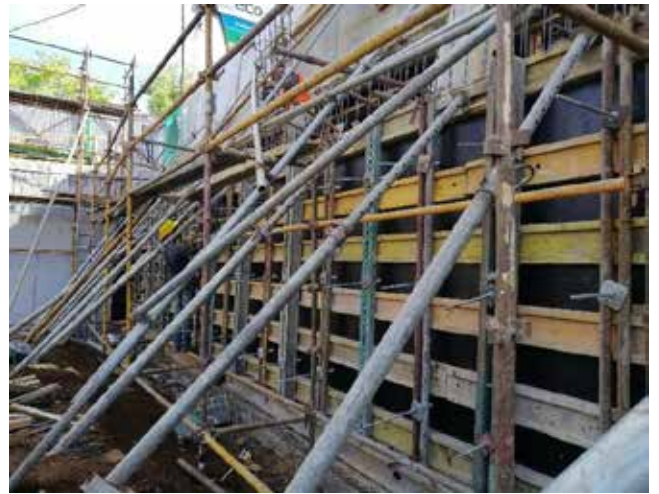
Photo 2: Shuttering to reinforcement of retaining wall along GL A-AX' |1'
