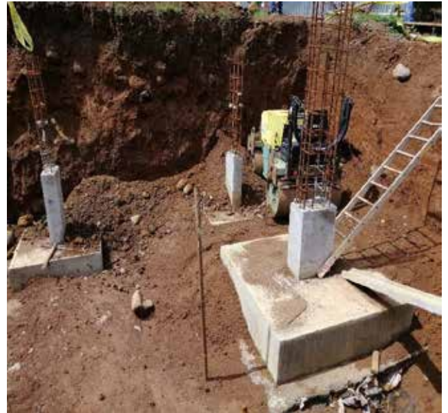
Photo 4: Backfilling at water tank area
