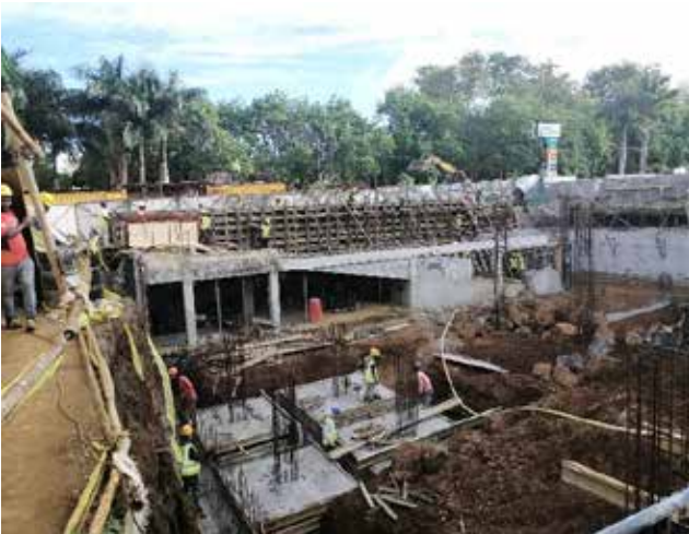
Photo 15: Deshuttering of column bases along GL B-C|2-3 and retaining wall along GL A'|1'-6
