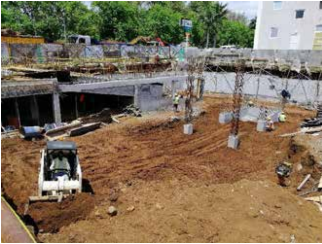
Photo 9: Backfilling and compaction along GL Ax'-C'
