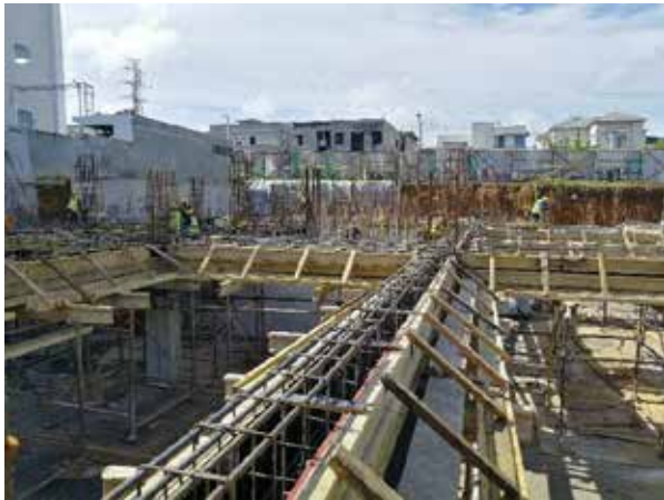
Photo 5: Shuttering to beam reinforcements along GL E-F|3
