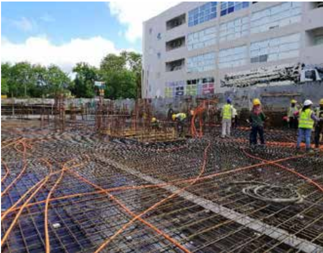
Photo 11: Reinforcement and conduits installation at soffit of Basement B1 floor slab
