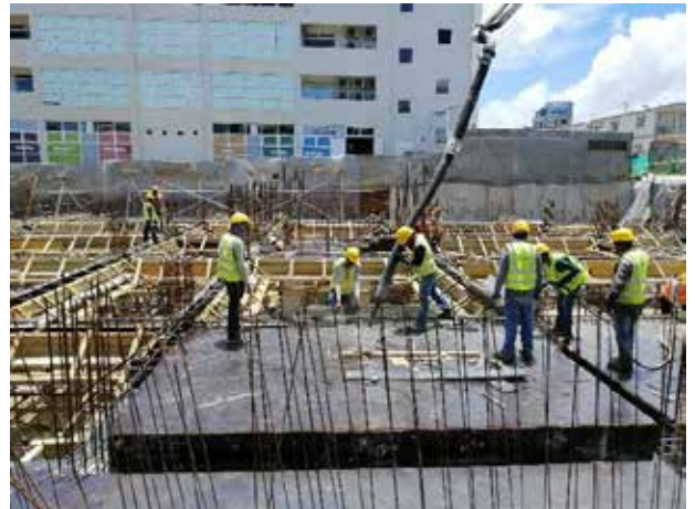
Photo 6: Casting of beam – GL G-H|5
