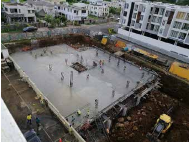
Photo 12: Casting of Basement B1 floor slab
