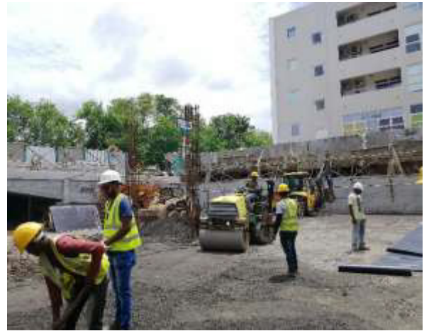
Photo 2: Compaction of crusher run along GL C-D|2-5
