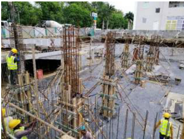
Photo 7: Shuttering to reinforcement of columns at GL B-C|1-6
