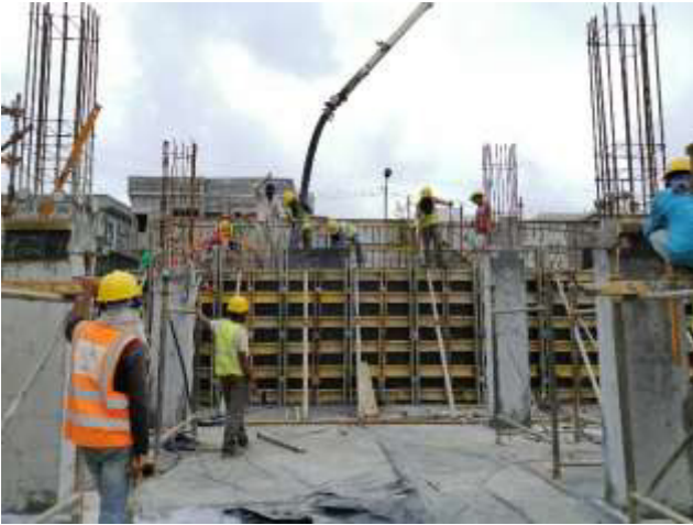
Photo 9: Casting of retaining wall along GL Kx|1-4
