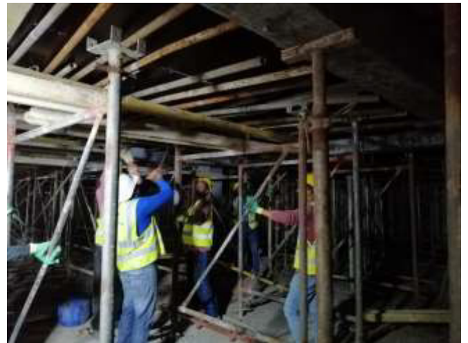
Photo 8: De-shuttering at soffit of Basement B1 floor slab
