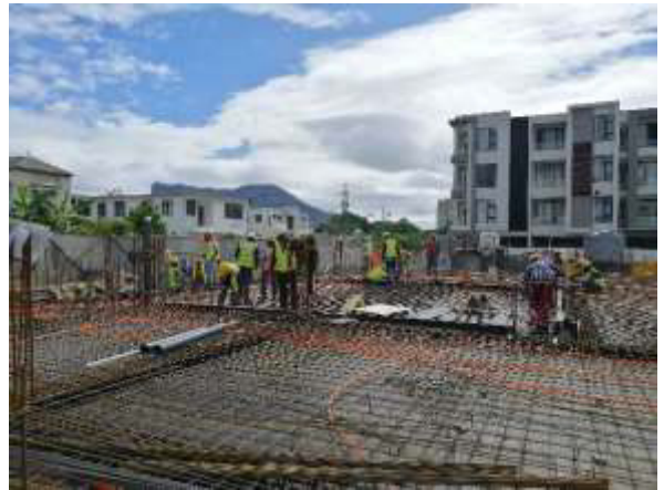
Photo 2: Reinforcement, fixation of conduits and sleeves to slab along GL H-Kx|3-7
