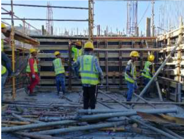
Photo 1: Shuttering to RC walls at water tank along GL J-Kx|4-7
