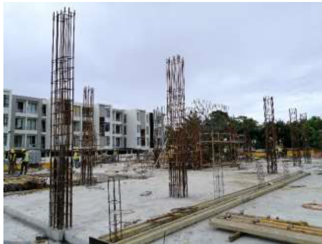
Photo 10: Column reinforcement for column extension on Ground Floor GL D-F|7
