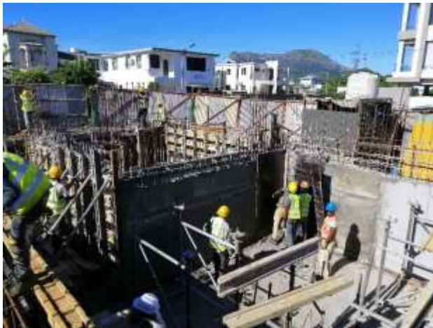
Photo 3: De-shuttering at water tank GL J-Kx|4-7
