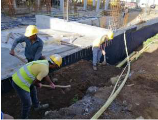
Photo 5: Backfilling at ramp along GL A'
