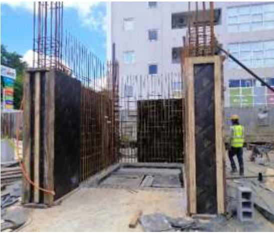
Photo 6: Shuttering to reinforcement at staircase along GL B-C|1-2
