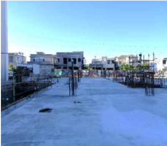
Photo 8: Casted Basement B1 slab/ Ground Floor
