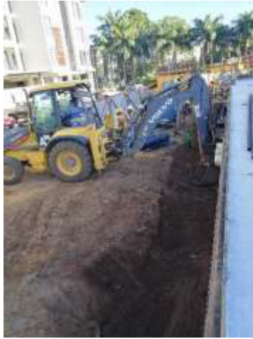
Photo 9: Backfilling along GL 7
