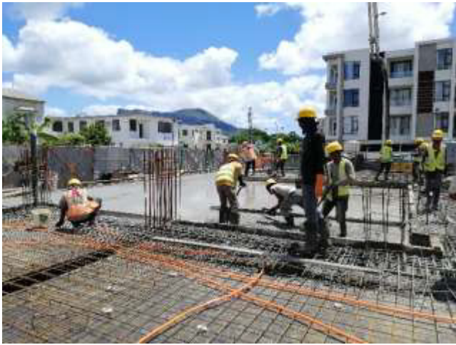
Photo 7: Casting of Basement B1 slab at GL H-Kx|1'-7
